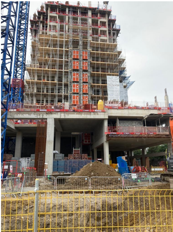
227-255 Ilderton Road under construction showing logistics space in the ground floor podium
