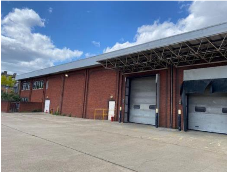
Tower Bridge Business Park south east facade
